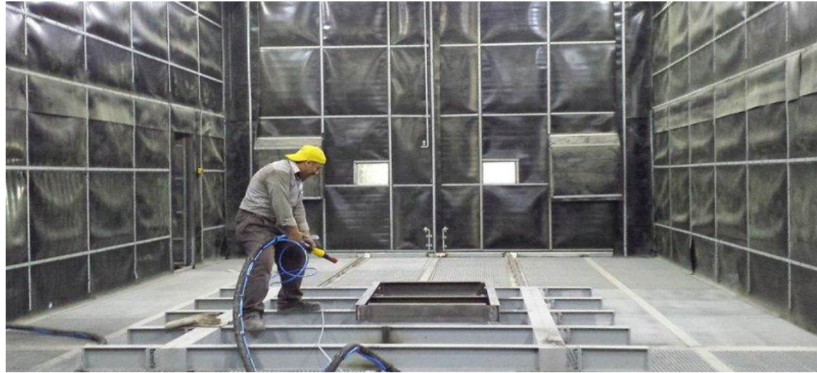
Manual blasting chambers
